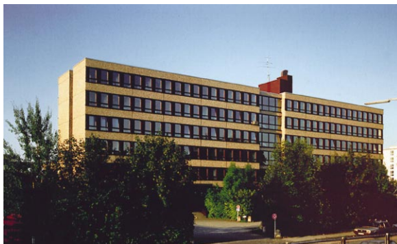
Branch Office, Perchtinger Strasse, Munich
